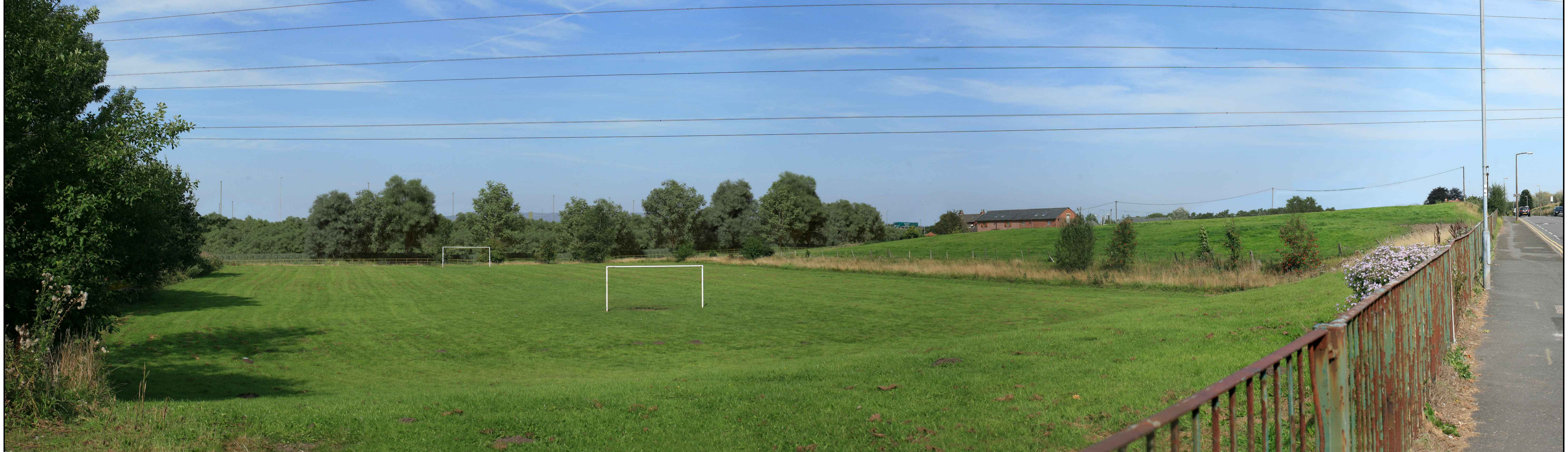
VIEWPOINT PM04: View looking north-east from Heywood Road near Parrenthorn High School to the new M60 west bound on-slip.
